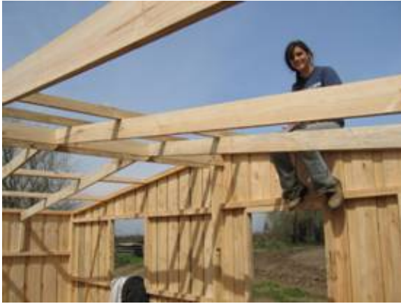
<left> Tere installing support beams for the roof.
